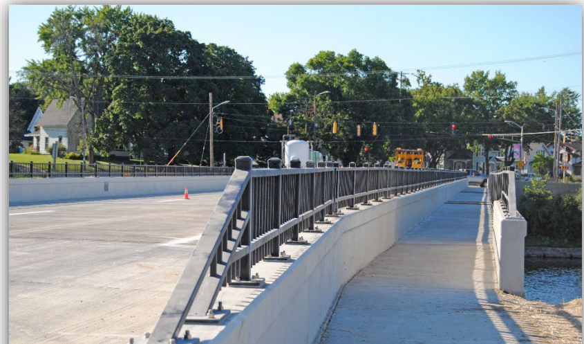
THE NEW PARAPET WALL ON THE ROBERT STREET BRIDGE IS SEEN AFTER COMPLETION OF CONSTRUCTION.
