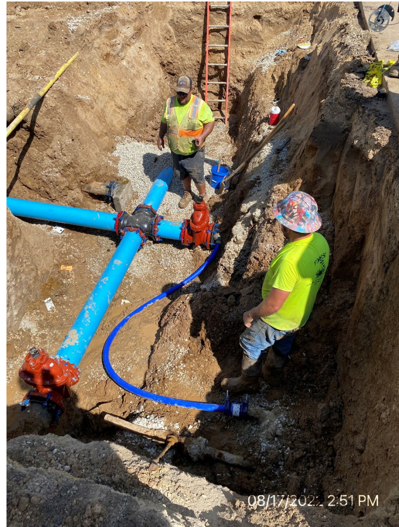
FOREST CONSTRUCTION WORKS ON THE WATER MAIN REPLACEMENT PROJECT IN AUGUST.
