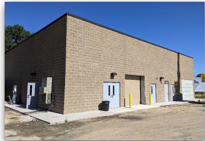
THE NEW WASTEWATER UTILITY BUILDING IS SEEN.
