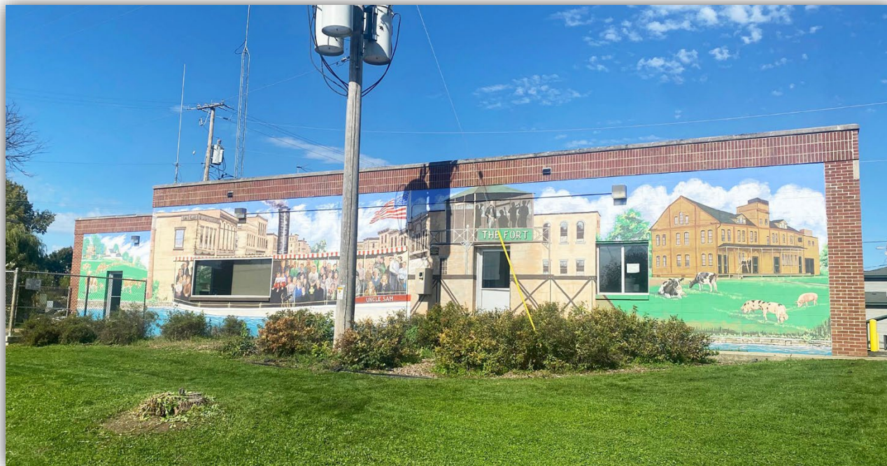
WATER UTILITY OFFICE ALONG THE ROCK RIVER INCLUDING FORT ATKINSON MURAL
